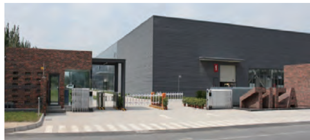
Tianjin factory Construction area of 30,000 square meters
